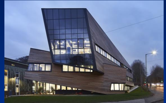
Ogden Centre West
